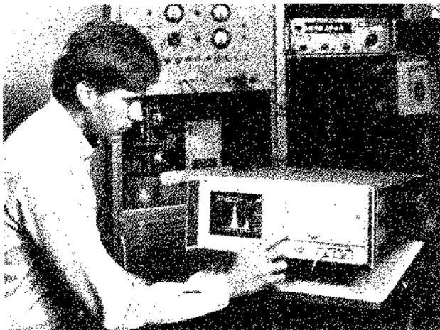
*Pulse width jitter, pulse-repetition frequency, and RF pulse rise time can be measured directly with the HP 5371A to simplify radar system characterization.*
